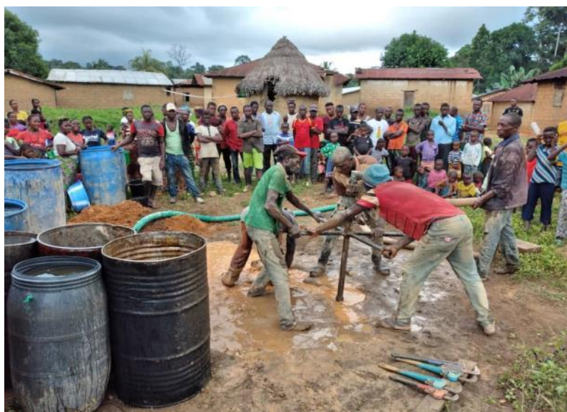
Manual borehole drilling in the village of Gbassadou, municipality of Fangamadou.
