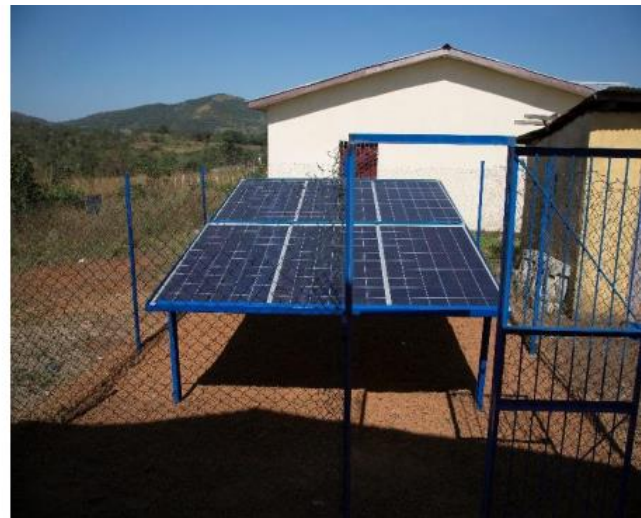
Top left: Water tank (15m3) installed in Niossomoridou. Top right: Water fountain with three water points in Niossomoridou. Above, left: PME team installs a solar pump on an existing borehole. Above, right: Photovoltaic panels (1.6 kw) used to power the solar pump.
