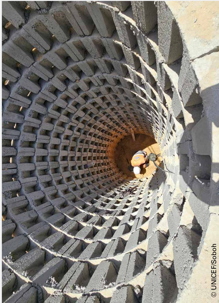
A septic tank is installed at Nasser Hospital in Khan Yunis in the southern Gaza Strip, State of Palestine, in June 2024.
